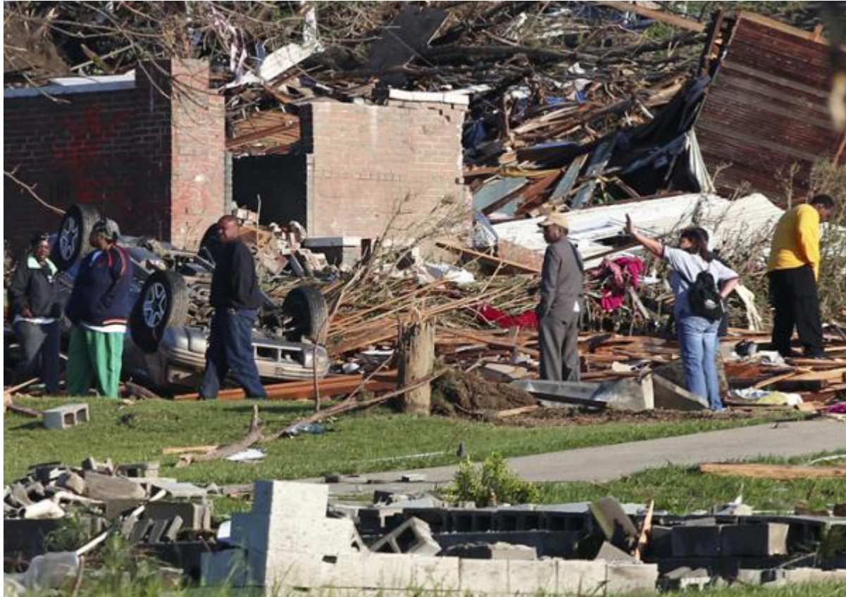
Residents inspect the aftermath of tornadoes that left this part of Pratt City, a suburb of Birmingham, Alabama, in ruins last Thursday. Picture: Reuters
